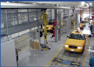
Bilprovningsanläggningen hos New York City Taxi and Limousine Commission i Woodside, Queens
